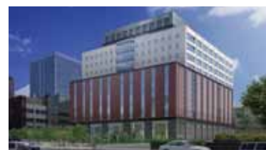
2012 Refurbishment of the IUHW Mita Hospital (Tokyo)
