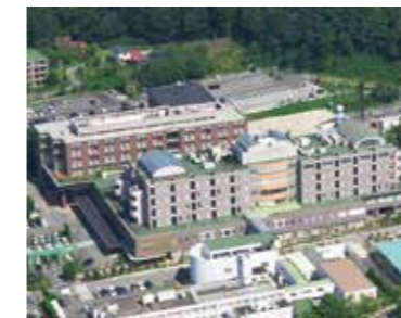
IUHW Hospital (Main Hospital)
